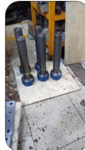
Cleaning the hydraulic cylinders
