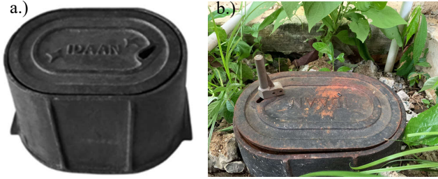
Fig. 5 Typical metal casing utilized in Panama City. (a) metal casing before installation. (b) a meter antenna protruding from metal casing after intervention.
