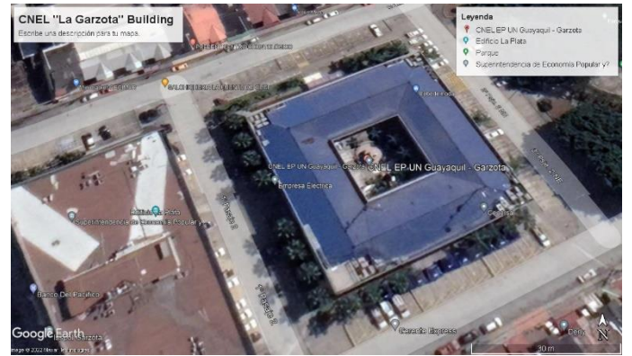
Fig. 1 Location of the Garzota building from Google Earth™
